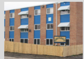
137 Avenue T South
