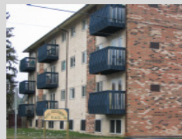
136 Avenue U South
